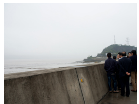
Qinshan NPP (Flood embankment)
